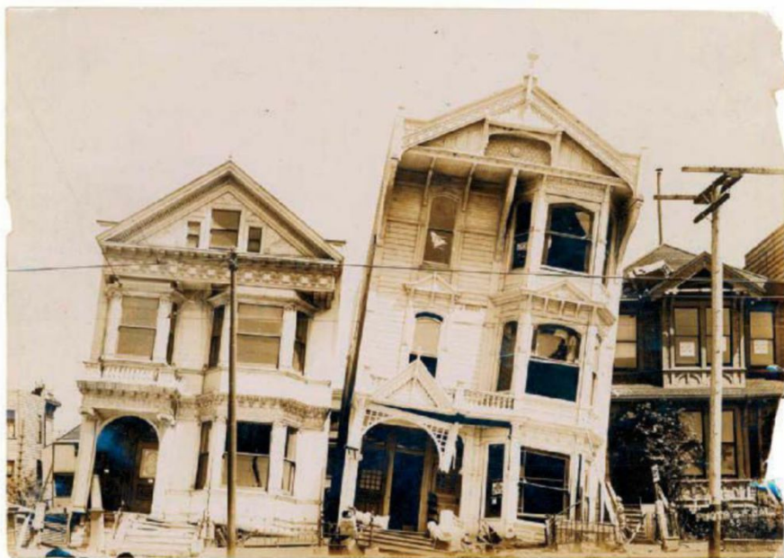
Houses in San Francisco, after an April 18, 1906, earthquake toppled them and killed thousands
