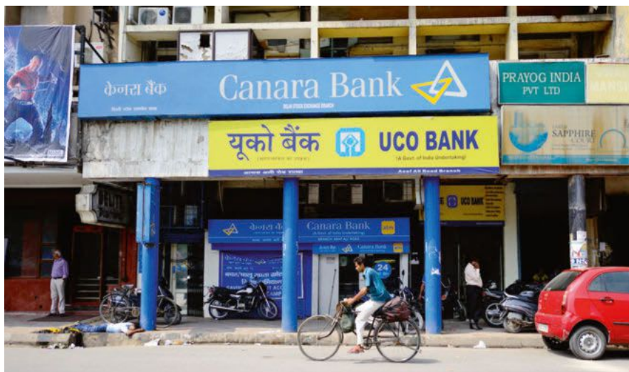
Pillars to be reinforced
