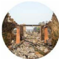
The devastating aftermath. They plan to rebuild.
