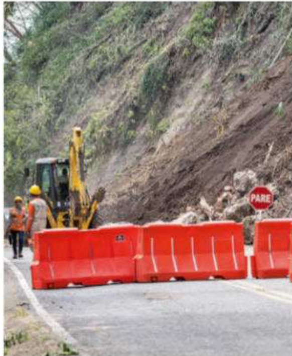
Removing road blocks
